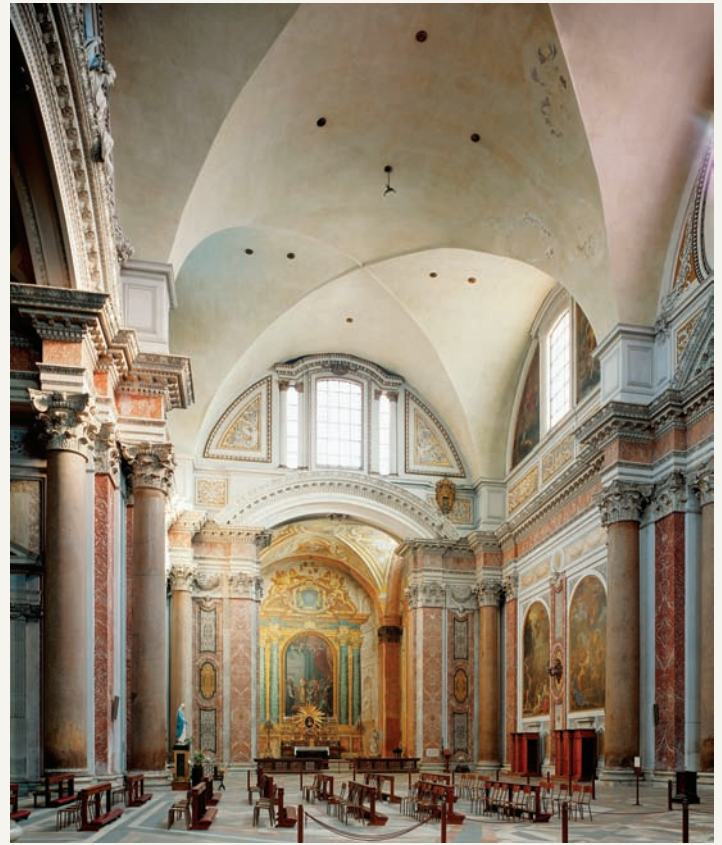
Roman hall with groin vaults (Baths of Diocletian, now Santa Maria degli Angeli, Rome, Italy, ca. 298–306)
